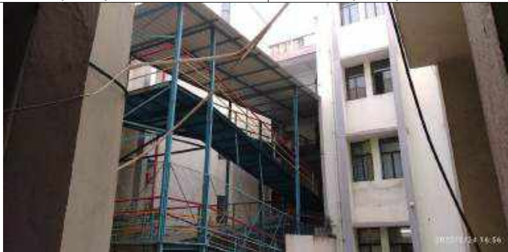
Ramp facility at C S E Block
