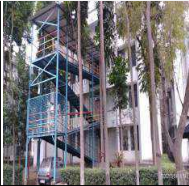
Ramp facility at Core Block
